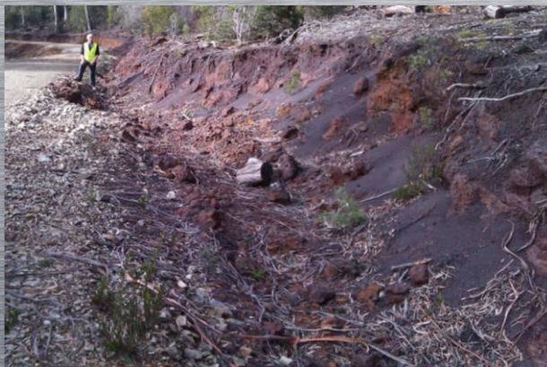
Riley DSO project surface deposits
