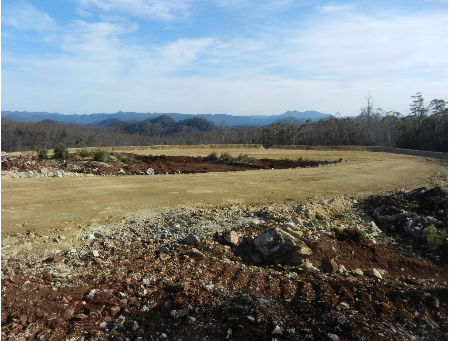
Figure 2: The ROM Pad at the Riley Iron Ore Project.
