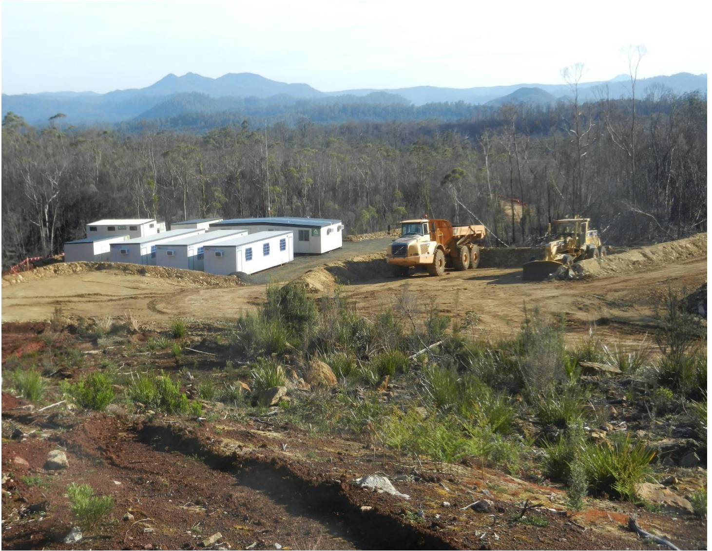
Figure 1: Establishing the site office at the Riley Iron Ore Project.
