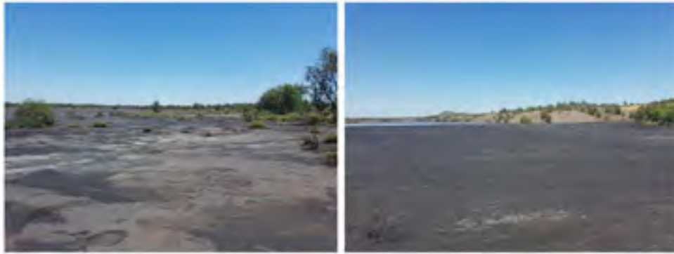
Figure 8.6: Original tailings dam (left) and Pit A tailings dam (right)
