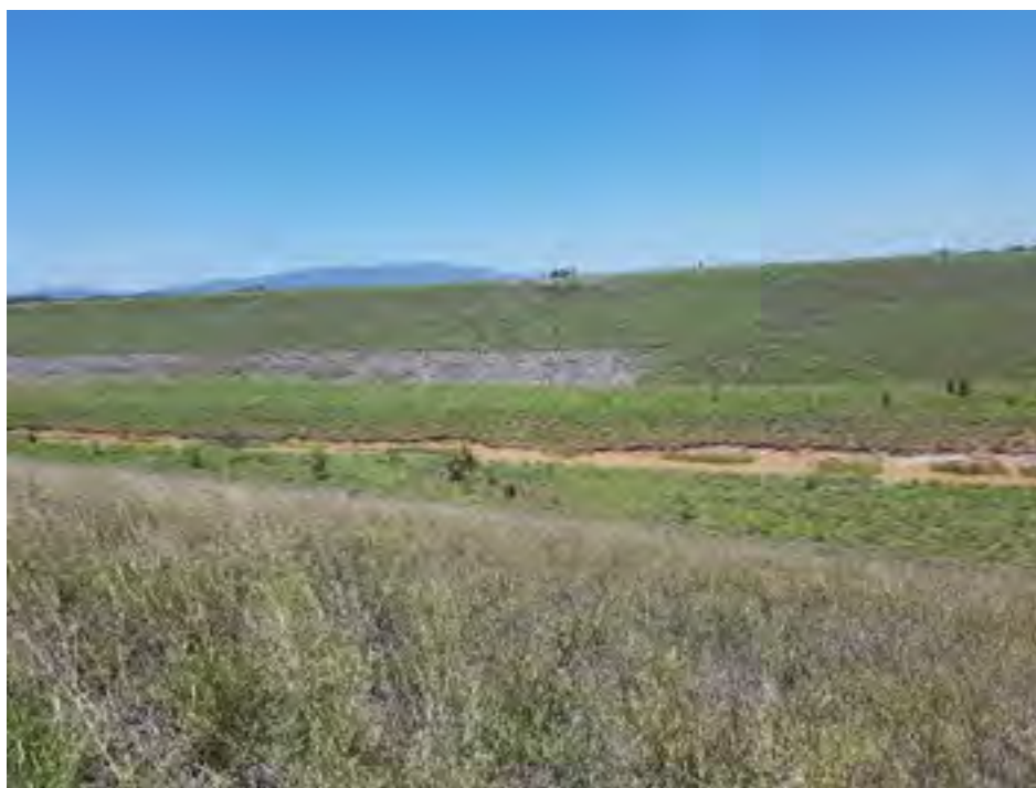
Figure 8.8: Blackwater Creek diversion
