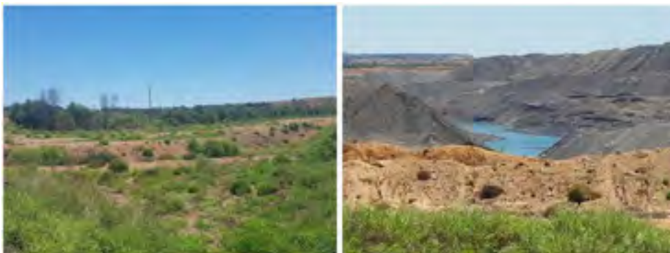
Figure 8.7: Pit A tailings discharge spillway (left) and Pit B tailings disposal facility (right)
