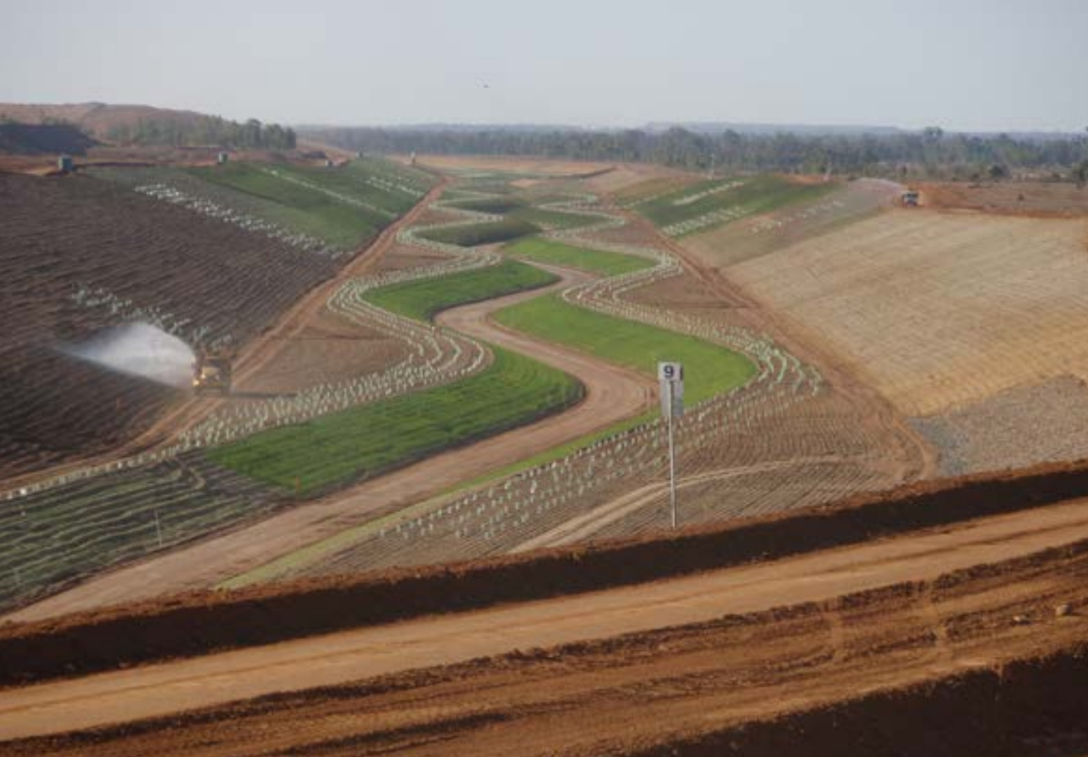
Above Blackwater Creek diversion, Curragh Mine
