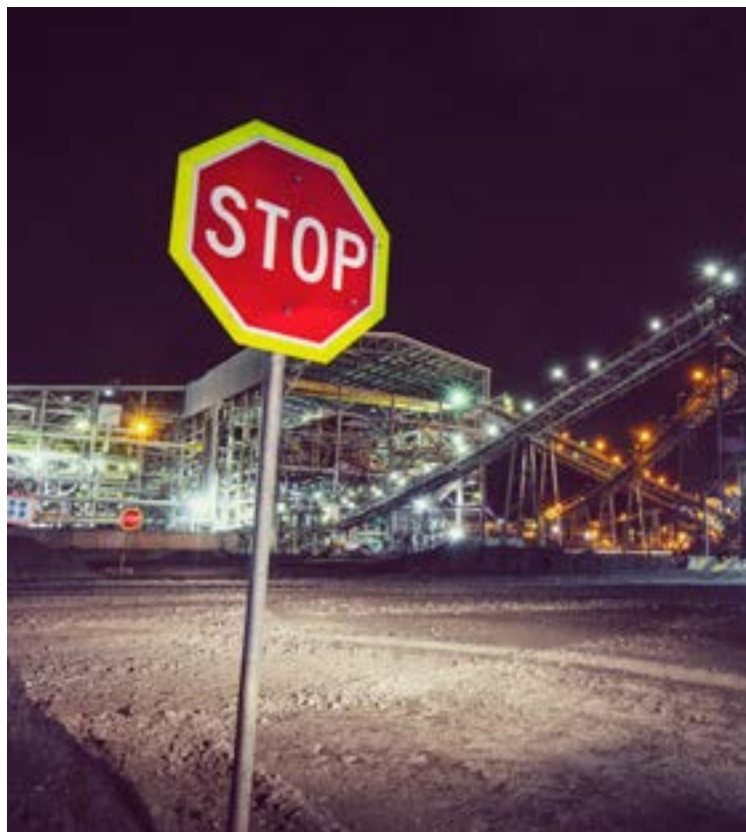
Below Coal Handling Preparation Plant, Curragh Mine
