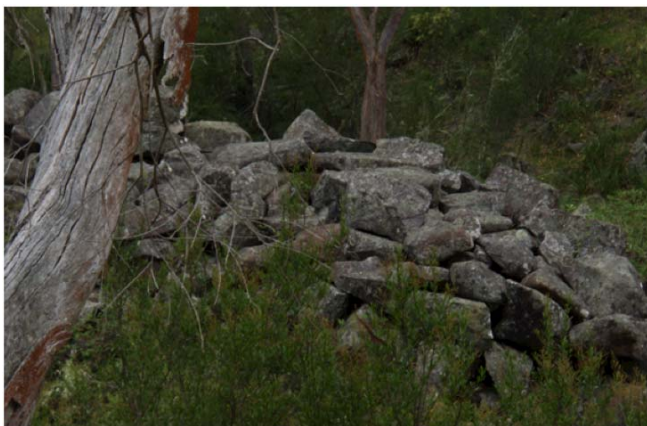
Stone wall with individual blasted blocks up to five tonnes that were hauled in 1863 by two man winch team from the basement of Kentucky Creek. A very rare feature in a 19 th century alluvial goldfield; the effort and resources expended is a testimony to richness of the gold along this portion of Kentucky Creek.
