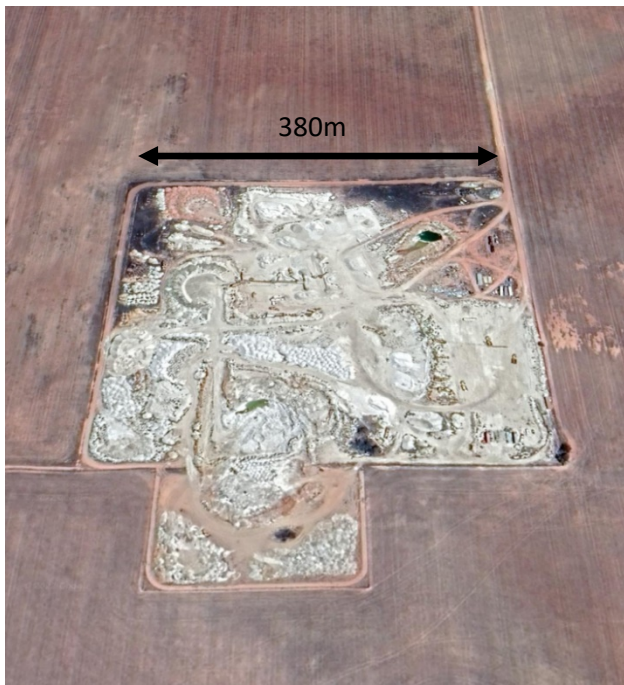
Figure 5: Cosh's North quarry within the Project
