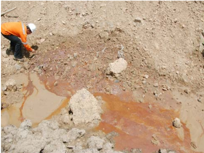
Road cutting oil seeps near NS-2 location
