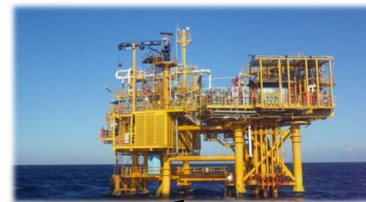
Existing Oyong pipeline to shore
