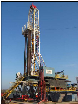
AD-1 Drilling Rig
