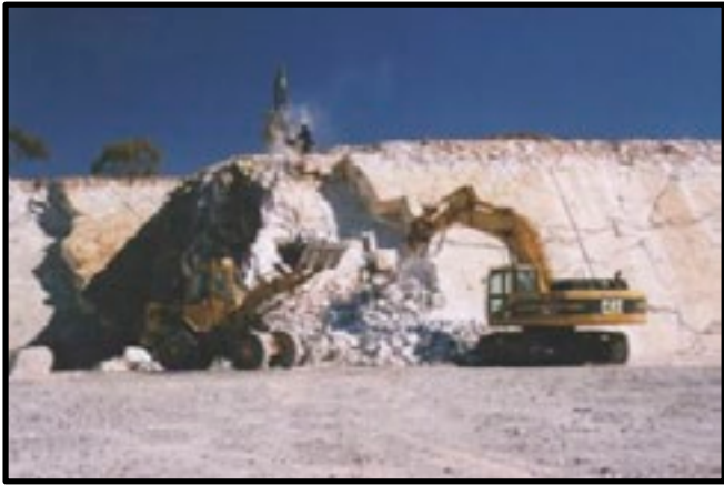
Plate 13: Excavator breaking ore from the face
