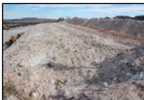
Plate 11: Top Soil and Weathered layer stripped
