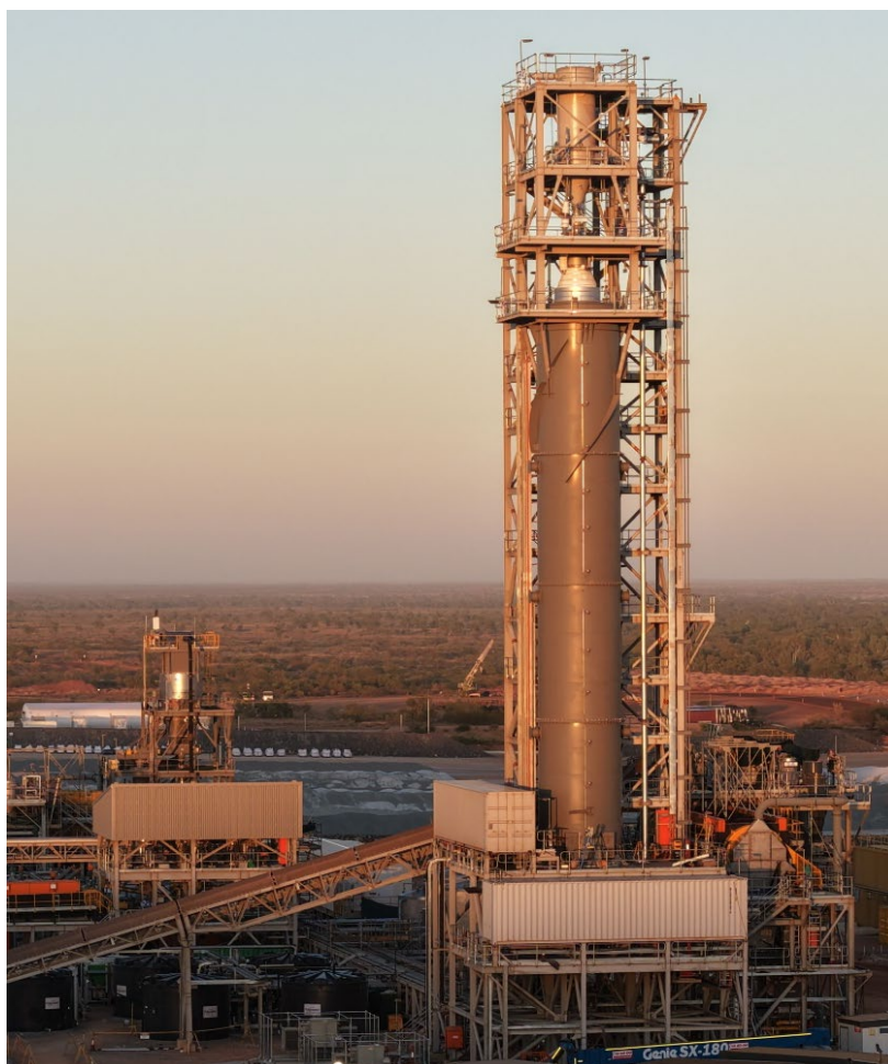
Figure 1. The completed Calix electric calciner at the PLS Pilgangoora Operation in Western Australia
