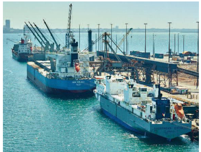
Figure 7 East Arm Wharf at Port Darwin.
