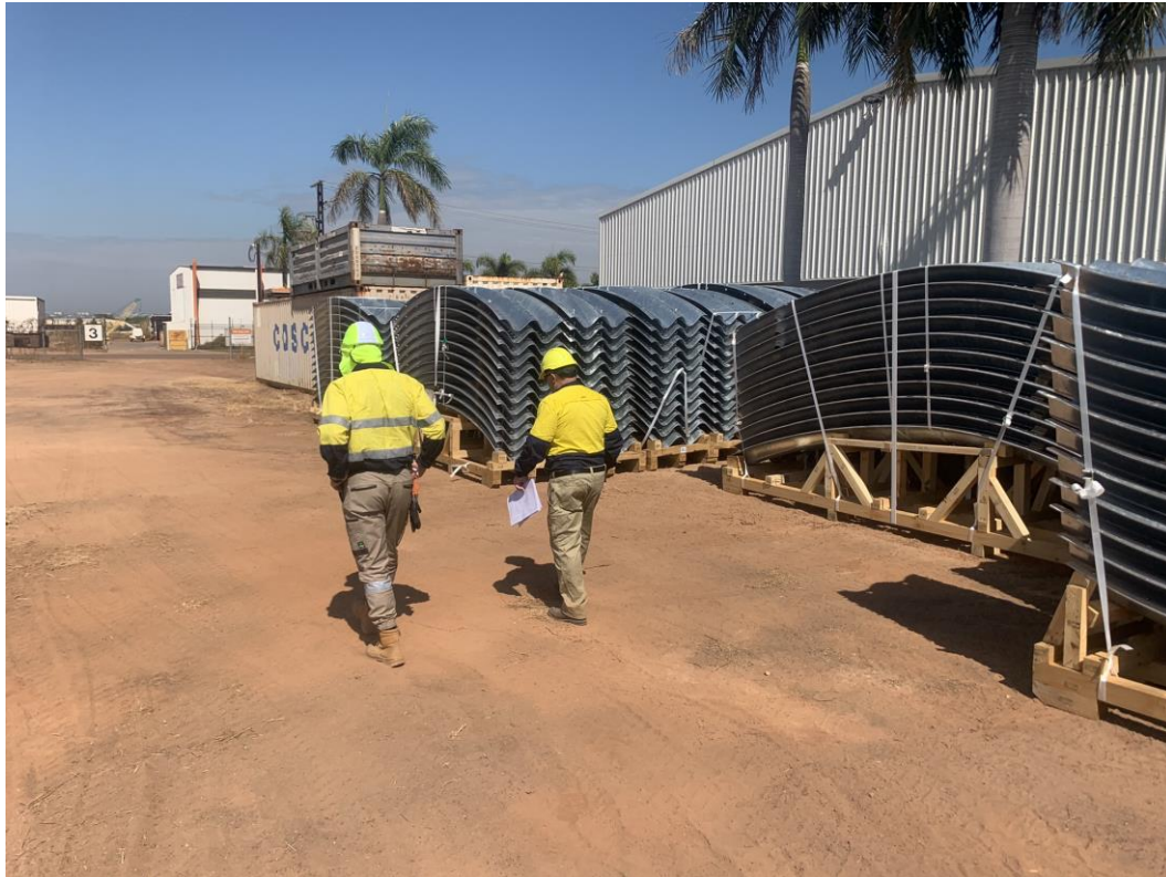
Tunnel liners delivered to Darwin laydown area
