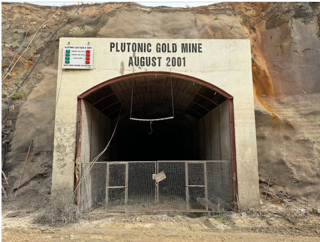
Figure 4: Plutonic East portal
