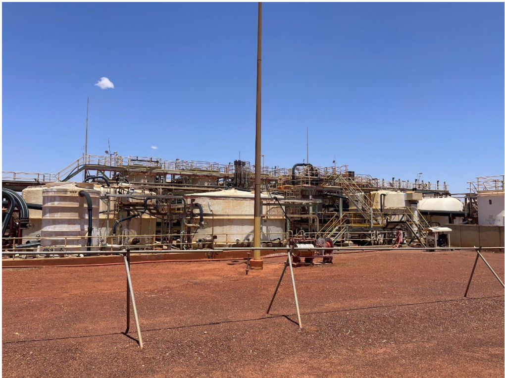
Figure 2-7: Solvent extraction plant
