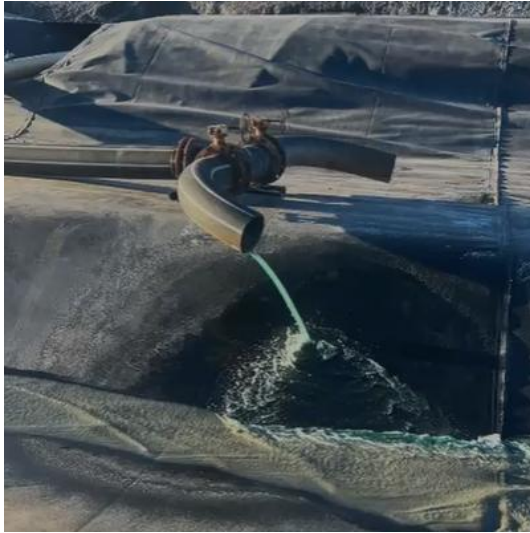
Off-flow piping discharging copper rich solution
