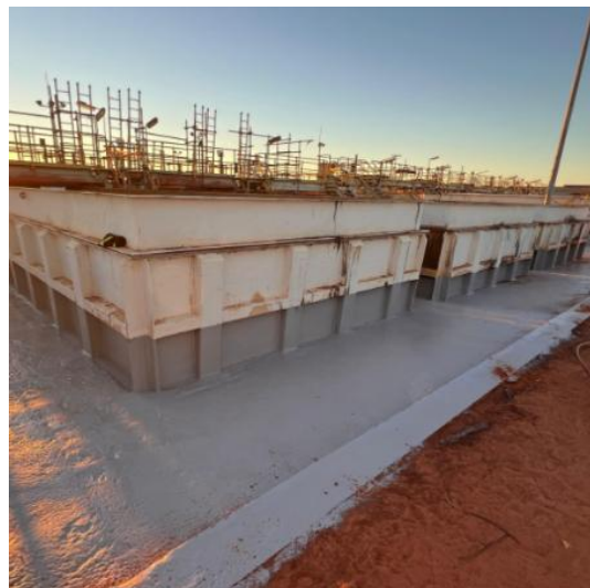
Acid proofing at mixer settlers complete
