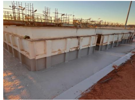
Acid proofing at mixer settlers complete
