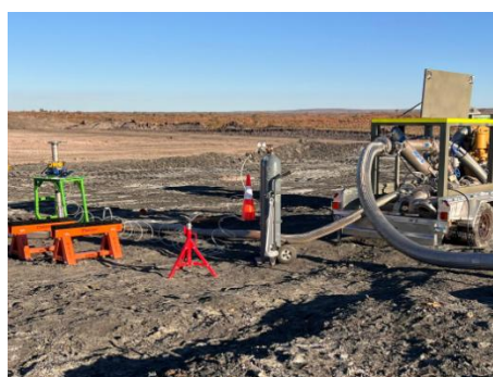
Testing direct injection leach system with water
