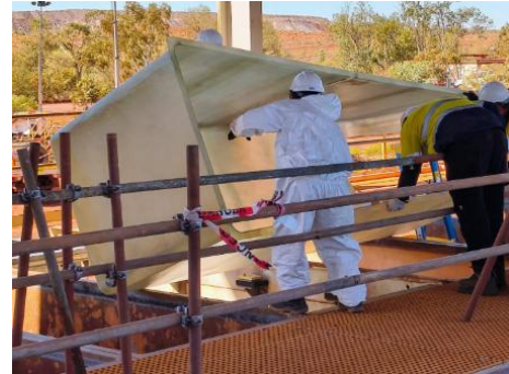
Installing fiberglass inserts for EW cells
