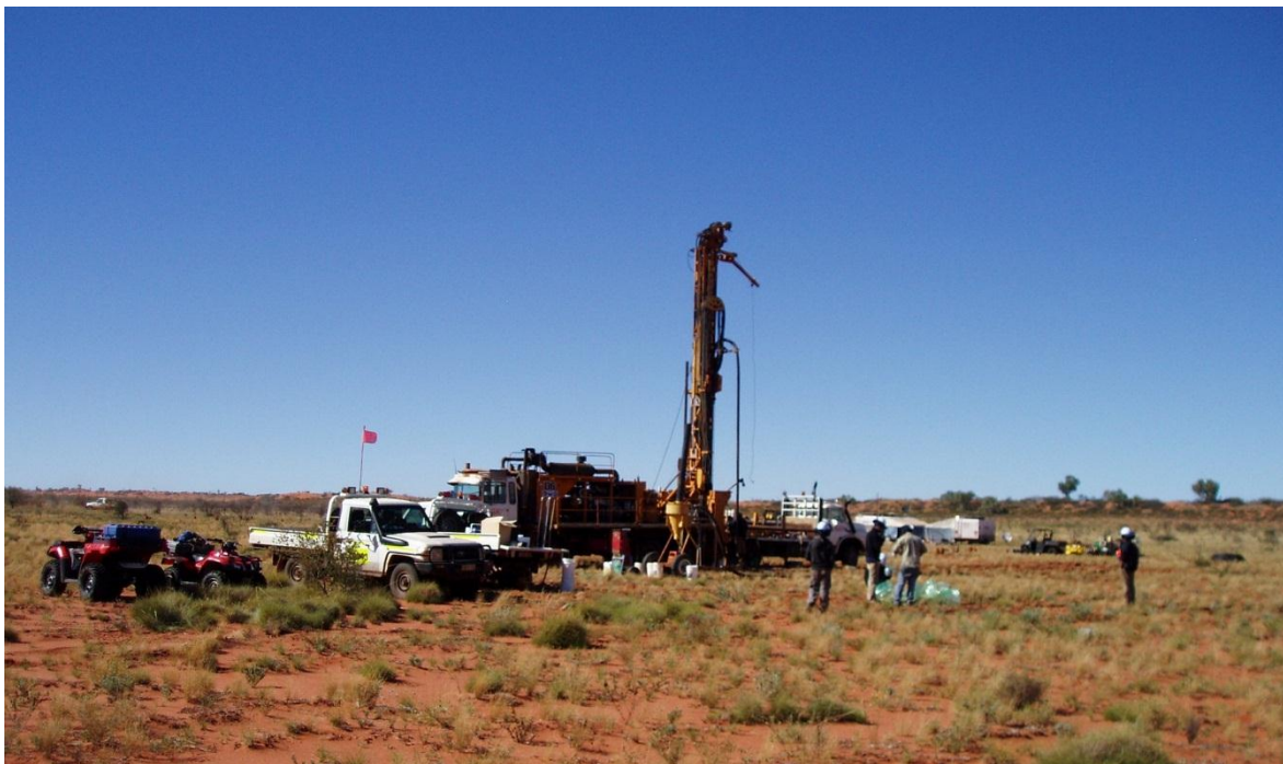
Drilling at Top Up Rise, Western Australia
