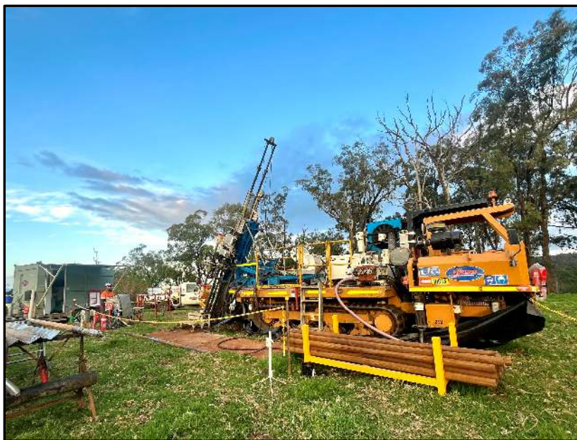
Figure 1 – May Queen – Drilling in progress at MQDD002
