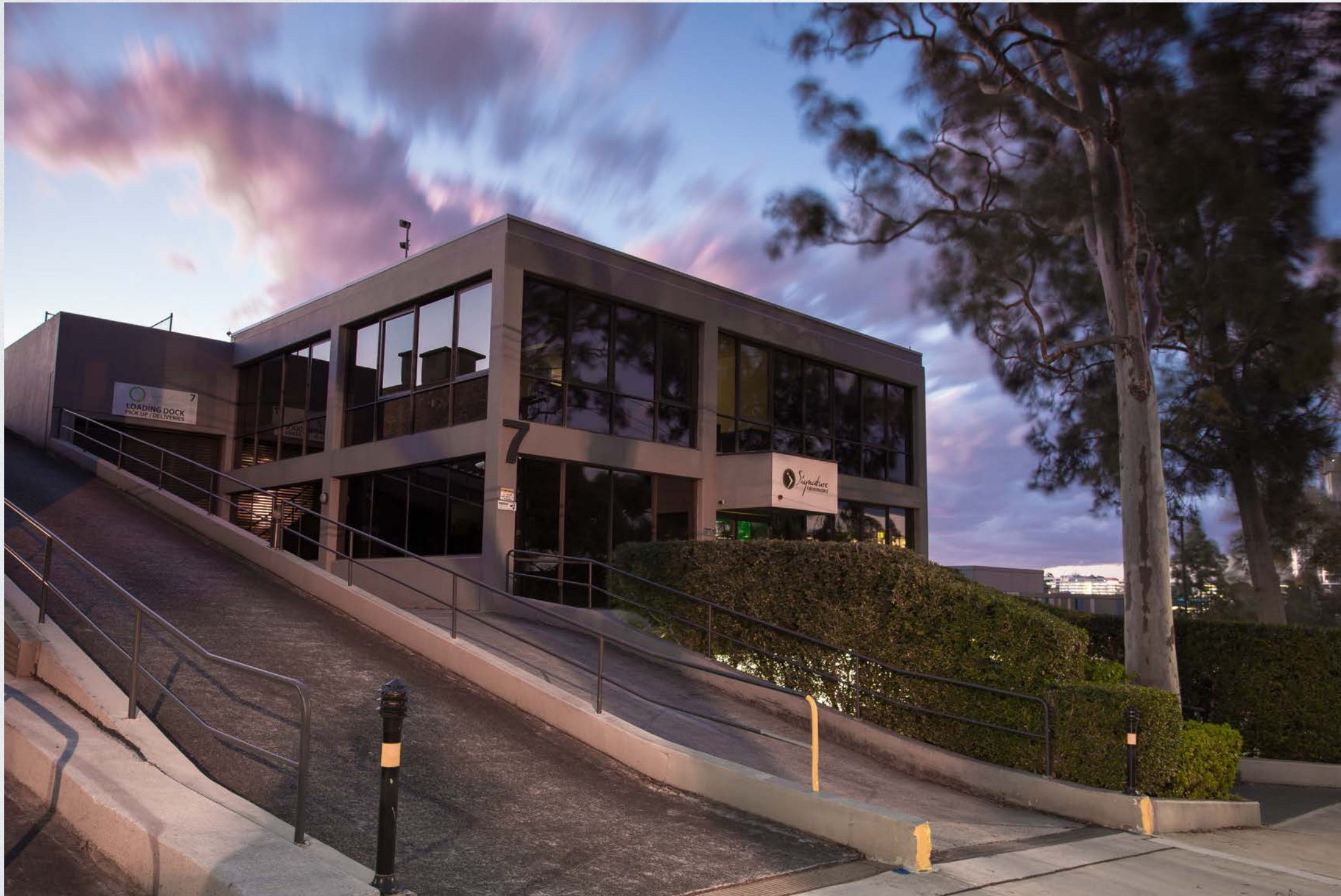
7 Sirius Road, LANE COVE NSW
