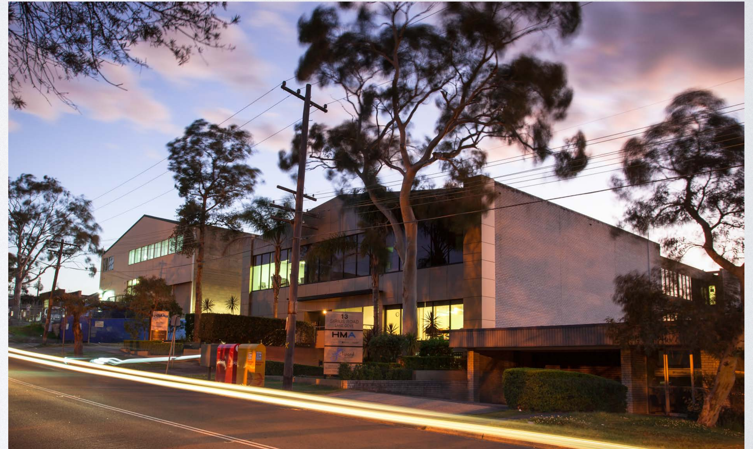
13 Sirius Road, LANE COVE NSW
