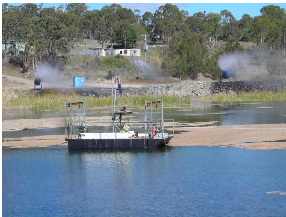
Figure 2: Drilling Pontoon on Shamrock Tailings Dam
