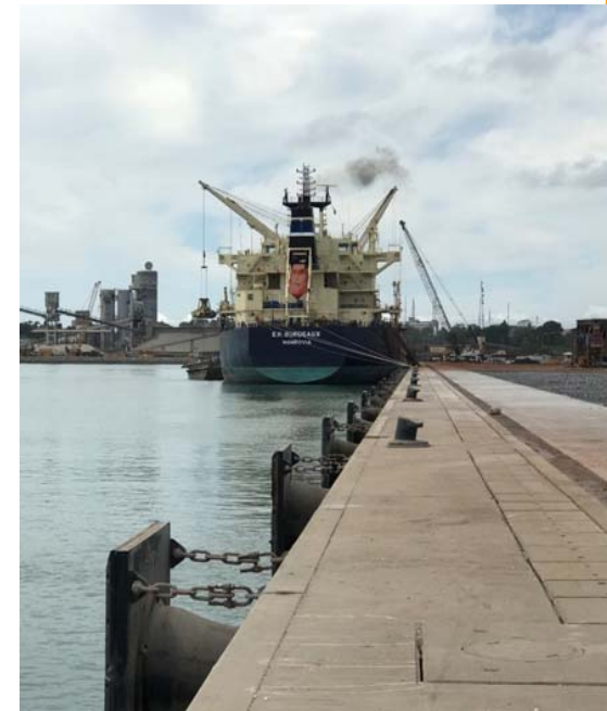
New 800m Dry Bulk jetty with 16m draft under construction
