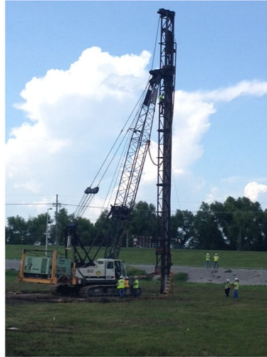
First pile being driven on site
