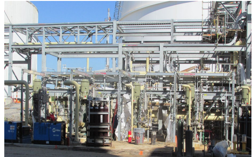
Ammonia loading pumps system being completed
