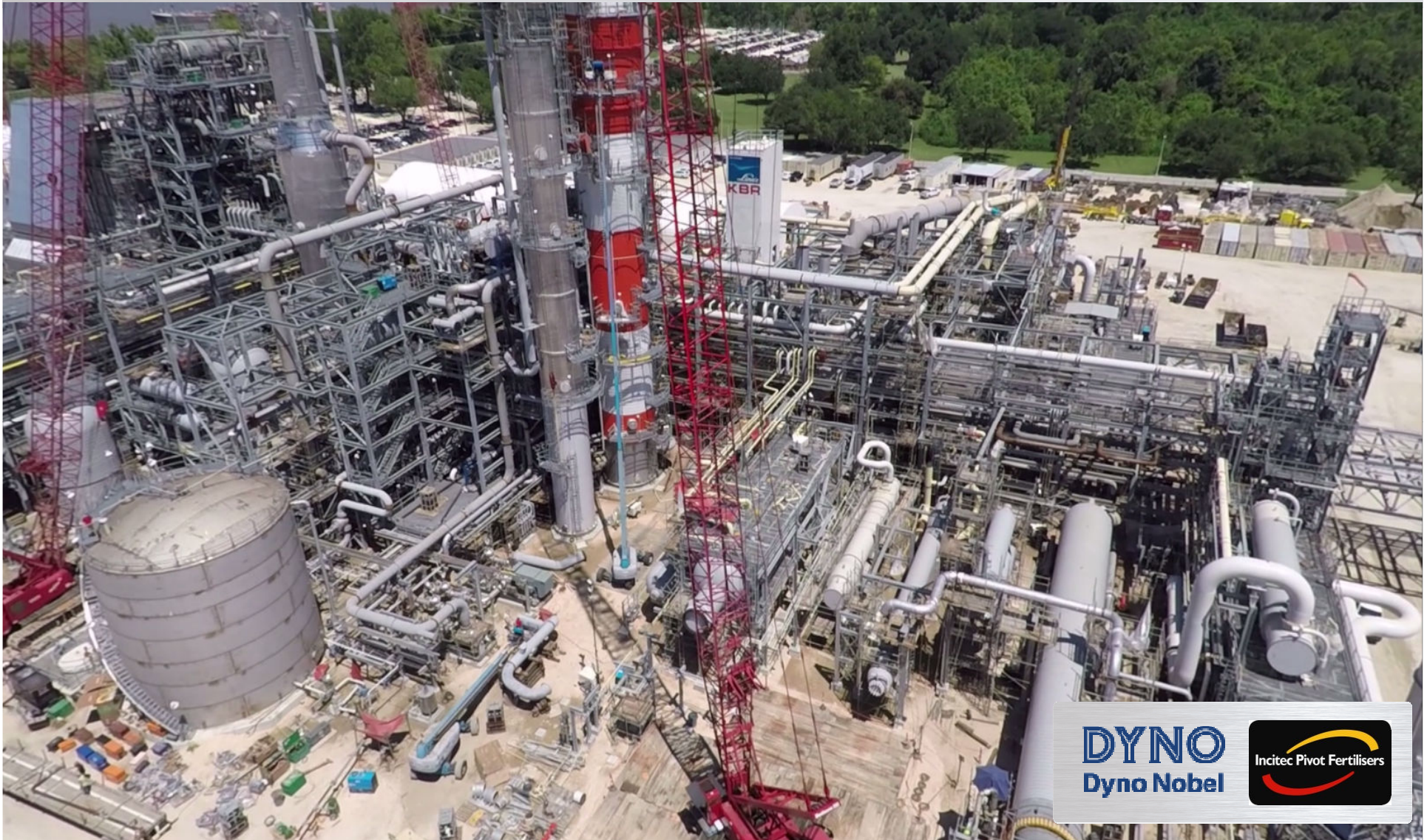
WALA ammonia plant under construction
