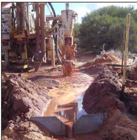
Cyclone Zircon Project – drilling for potential water supplies
