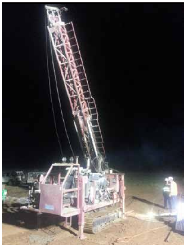
Clermont Project – Night diamond core drilling
