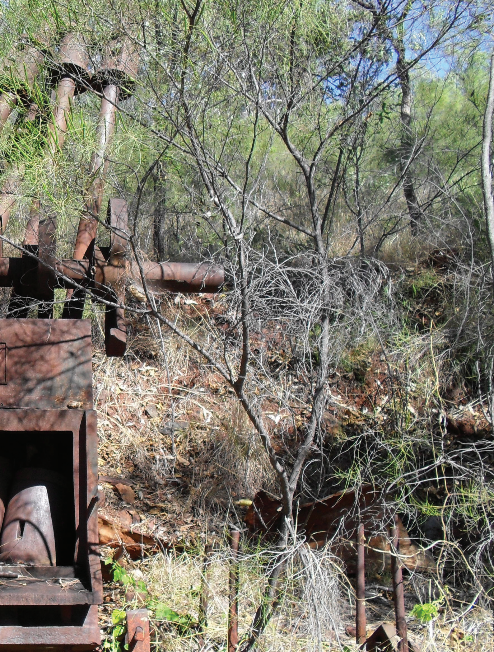
Gilbert River Project, North Queensland – Historic Battery Stamp
