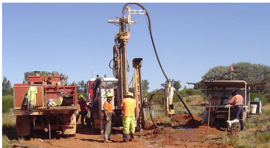
Test drilling for shallow water supplies – Cyclone, 2012
