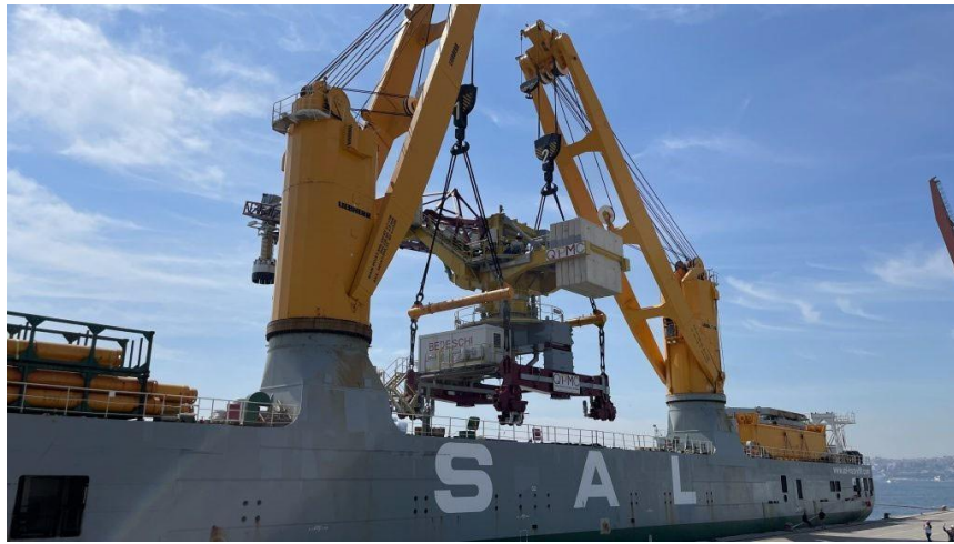
Figure 37: HLS lifting a fully assembled shiploader
