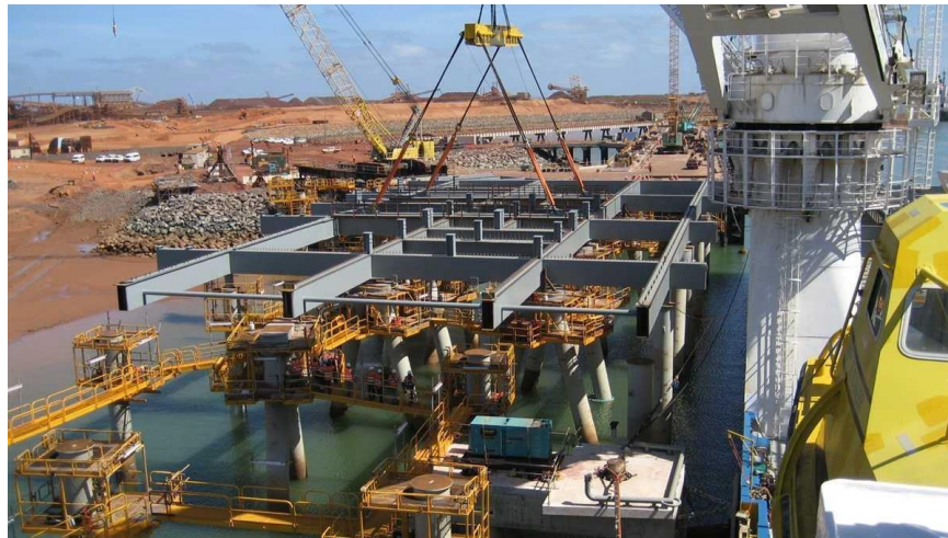
Figure 32: HLS installing prefabricated deck modules
