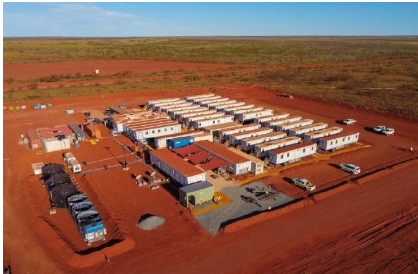
Figure 25: Typical construction camp using transportable buildings
