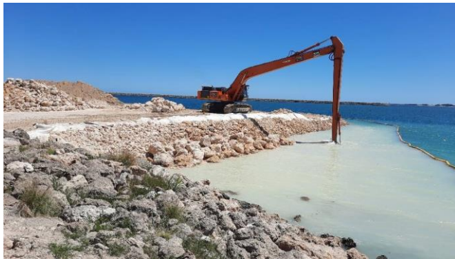
Figure 17: Installation of geofabric on top of fill
