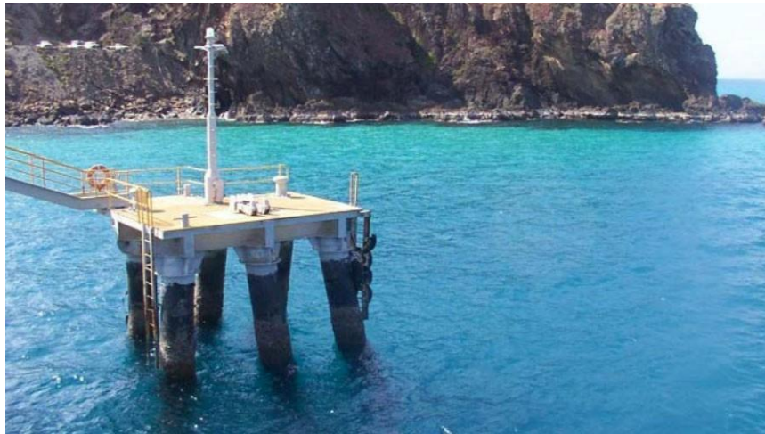
Figure 30: Mooring dolphin structure consisting of 6 raked piles
