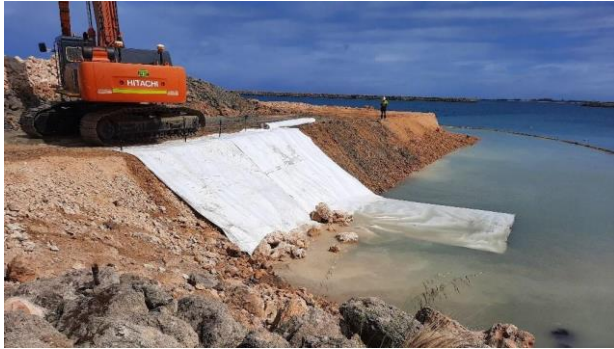
Figure 16: Installation of geofabric on top of fill
