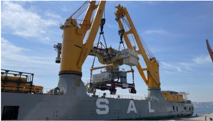
Figure 3637: HLS lifting a fully assembled shiploader
