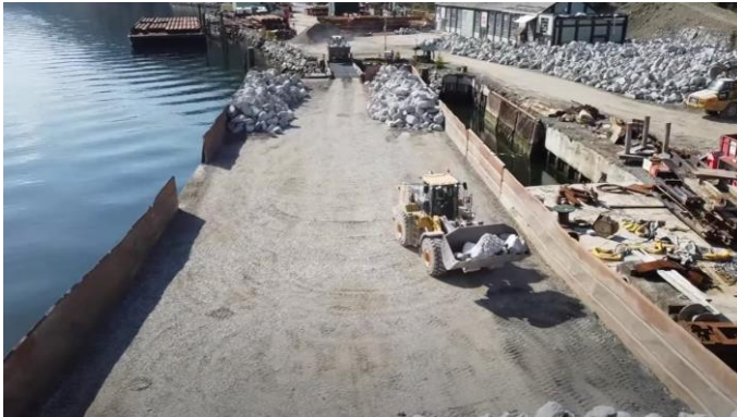
Figure 1314: Typical rock barge being loaded by front-end loader
