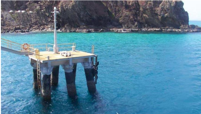
Figure 2930: Mooring dolphin structure consisting of 6 raked piles
