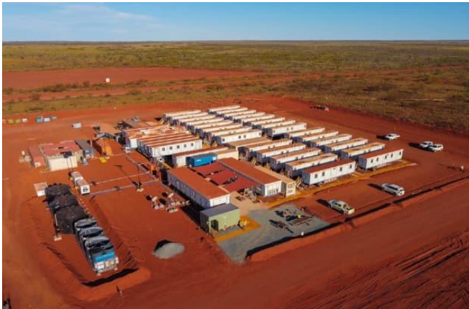
Figure 2425: Typical construction camp using transportable buildings
