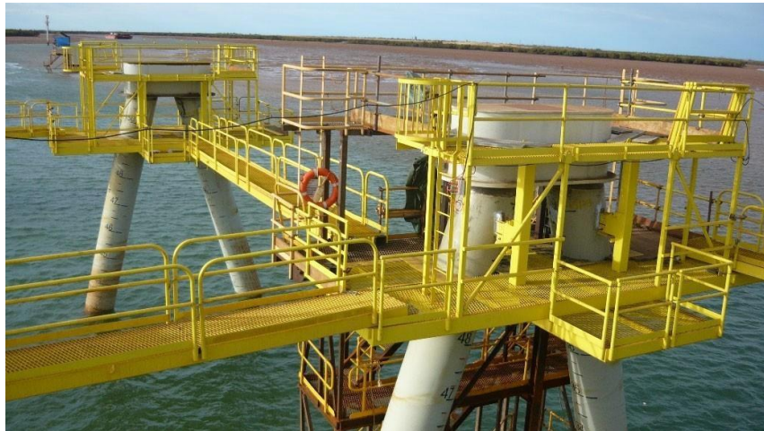
Figure 29: Pile bracing and walkways installed
