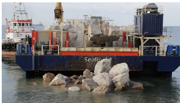
Figure 4.15: Typical rock barge being offloaded by front-end loader
