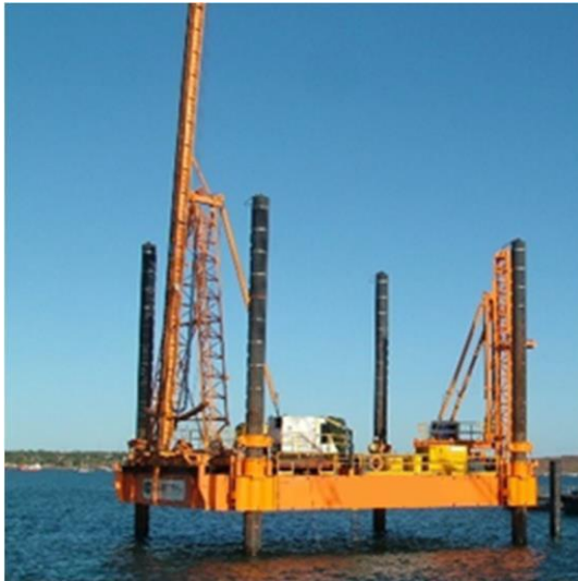
Figure 21: SEMP used to install mooring piles.
