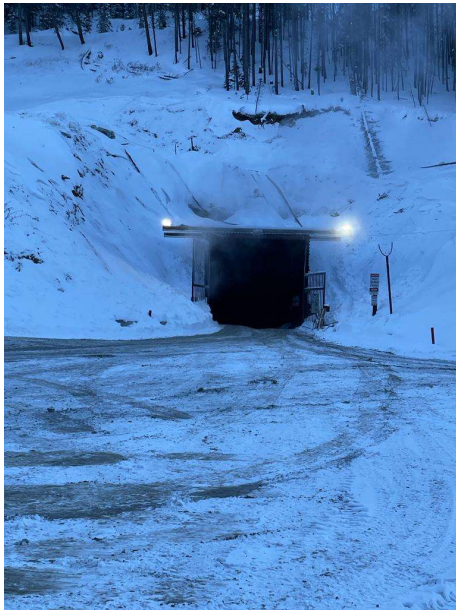
Figure 2 Portal at 10,000ft RL
