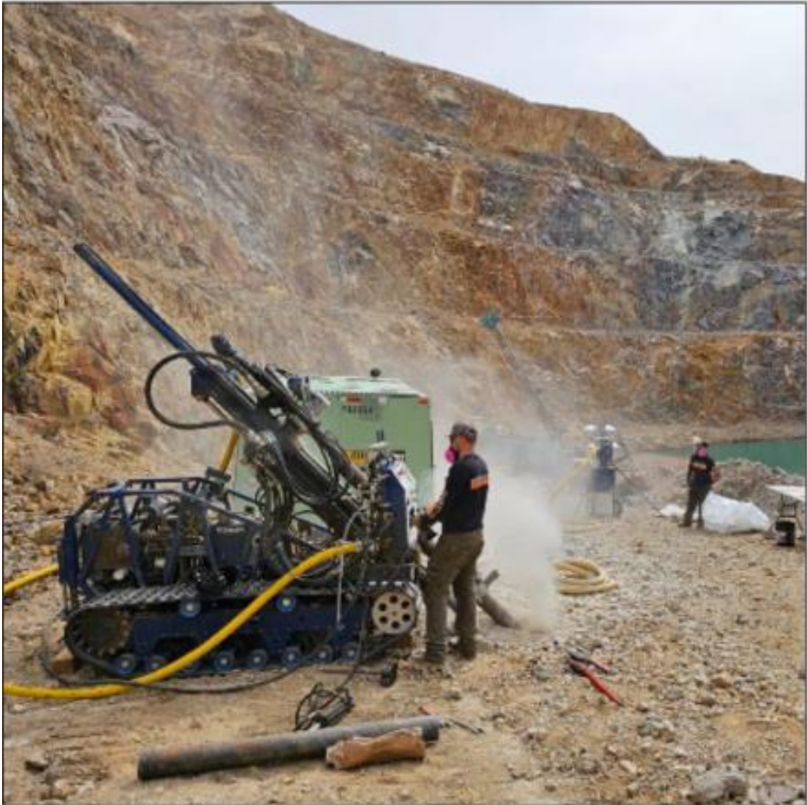
Figure 2 Company owned RC rig and compressor conducting infill drilling
