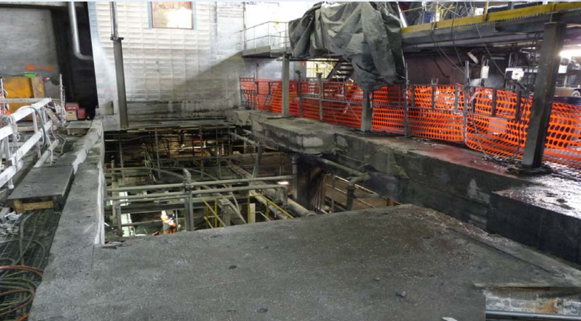
Concrete cutting for new filter position
