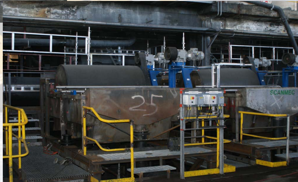
New magnetic separators 80% complete
