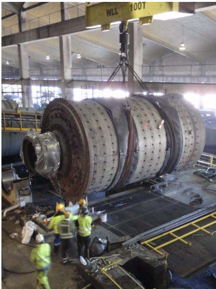
Figure 3 - additional secondary mill being lowered into position in June
