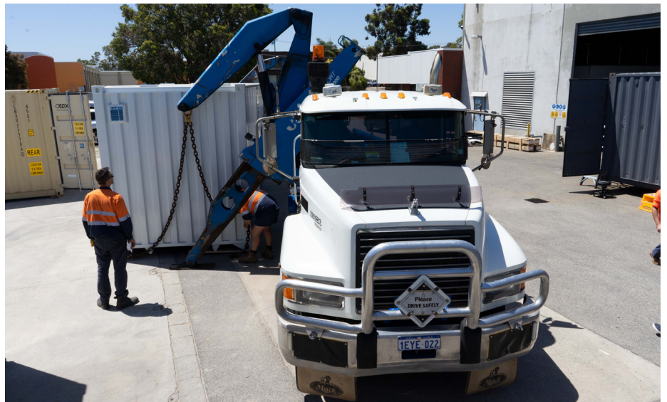
Road, rail or sea our modules are designed to travel. Cross Connect Room 1 will provide our clients with bespoke solutions and unprecedented telecommunications choices.
