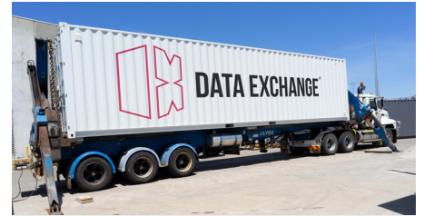
Telecom Module or Cross Connection Room
