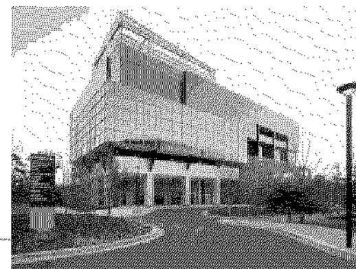
Building C, 11 Talavera Road, North Ryde
