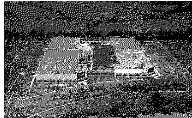
Beaumeade Telecom - Beaumeade Circle, Ashburn, Virginia
