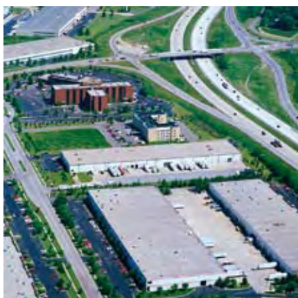
1825 Airport Exchange Boulevard, Erlanger, Kentucky
