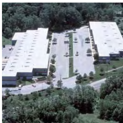
1015 & 1025 West Nursery Road, Linthicum Heights, Maryland
