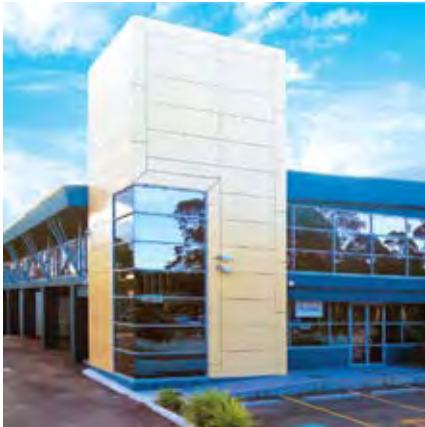
145-151 Arthur Street, Flemington, NSW
