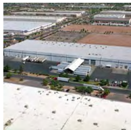
431 North 47th Avenue, Phoenix, Arizona
