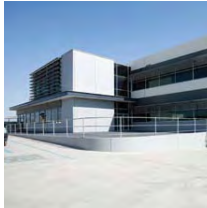
12-18 Distribution Drive, Laverton North, VIC
