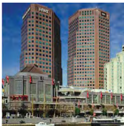
Southgate Complex, 3 Southgate Avenue, Southbank, VIC
