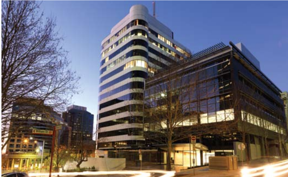
Victoria Cross, 60 Miller Street, North Sydney, NSW, showing the newly developed building
