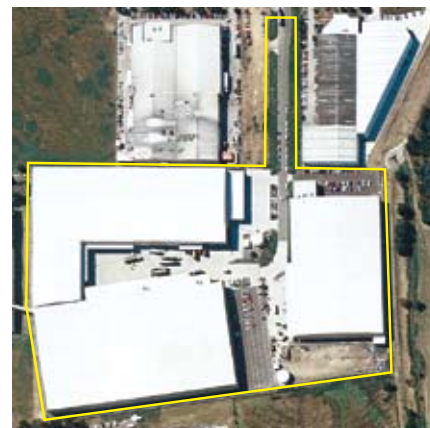
Knoxfield Industrial Estate, Henderson Road, Knoxfield, VIC
