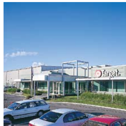
Target Distribution Centre, Tarras Road, Altona North, VIC
