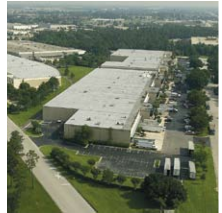
Orlando Central Park, 7600 Kingspointe Parkway, 8259 Exchange Drive, 7451-7488 Brokerage Drive, 2900-2901 Titan Row, Orlando, Florida
