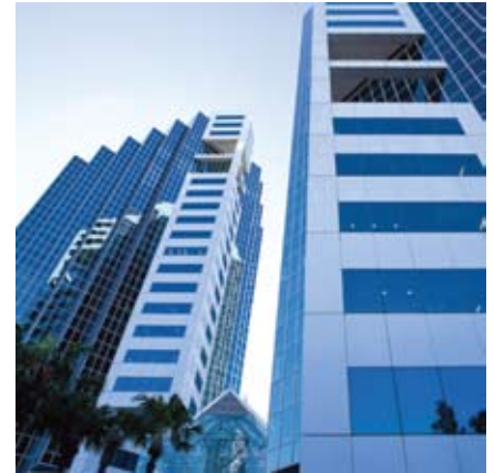
The Zenith, 821 Pacific Highway, Chatswood, NSW
