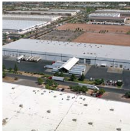
431 North 47th Avenue, Phoenix, Arizona
