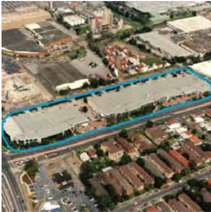
79-99 St Hilliers Road, Auburn
