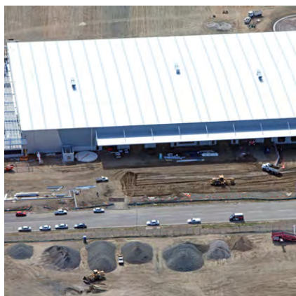
Quarry Industrial Estate, 2 Bellevue Circuit, Greystanes
