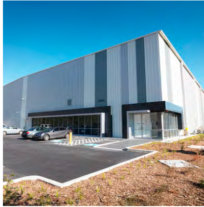
Quarry Industrial Estate, 5 Basalt Road, Greystanes
