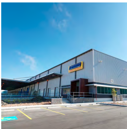
Quarry Industrial Estate, 2-6 Basalt Road, Greystanes
