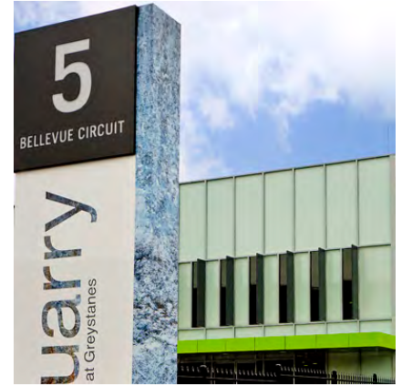
Quarry Industrial Estate, 5 Bellevue Circuit, Greystanes
