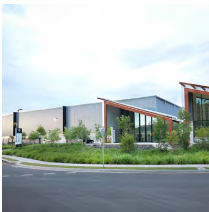
Quarry Industrial Estate, 8 Basalt Road, Greystanes
