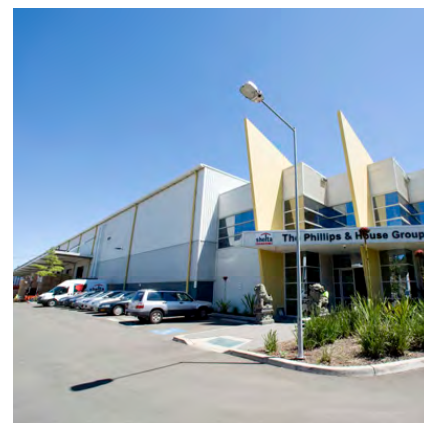
1 Foundation Place, Greystanes
