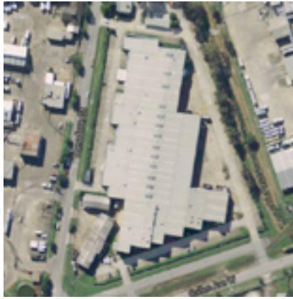
112 Cullen Avenue, Eagle Farm
