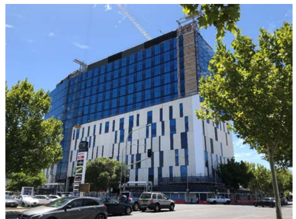
Calvary Adelaide Hospital – under construction.
