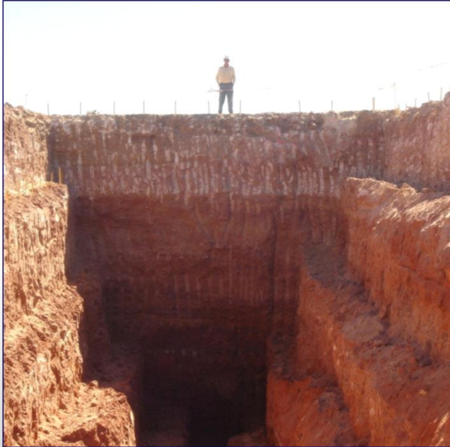
Trench for Bulk Sample
