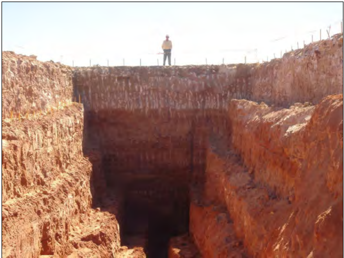
Figure 15 Tubas Red Sand final trench profile
