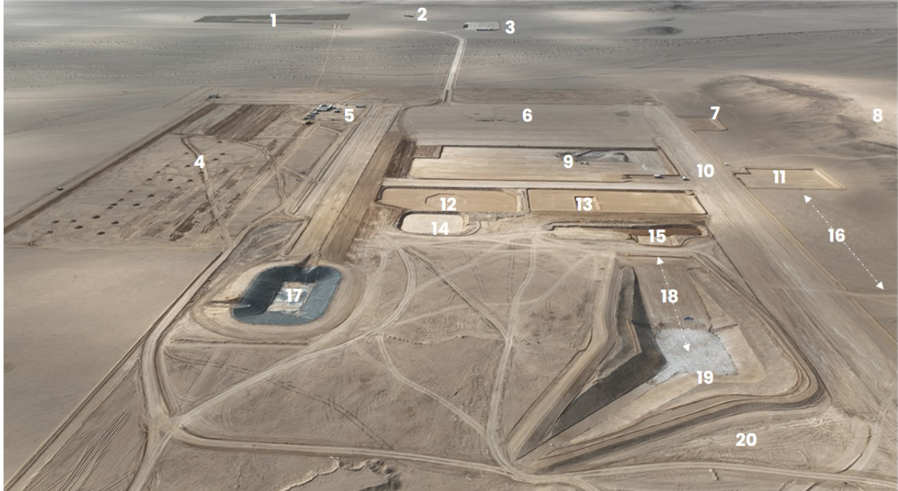
Figure 2: Aerial view of the Tumas bulk earthworks, May 2026.
