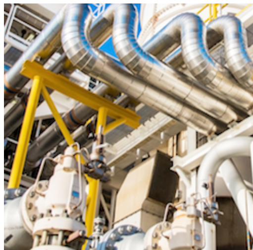
DEVELOPING INNOVATIVE, NOVEL PROCESS TO PURIFY ORE TO >99.7%
