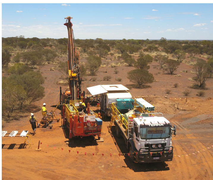
Figure 3: Diamond Drilling at Butcherbird February 2019.
