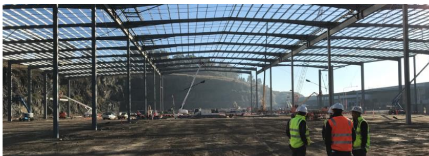
Construction progress: new Sydney Contract Logistics facility
