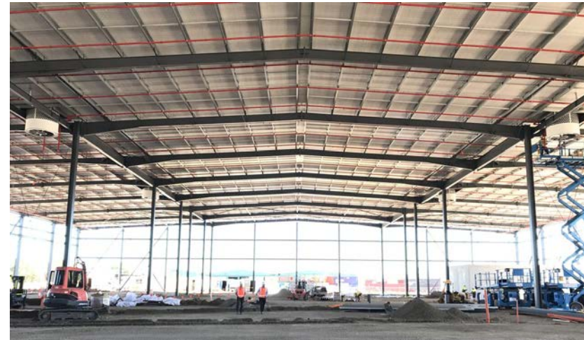
Construction progress: new Brisbane wholesale distribution centre
