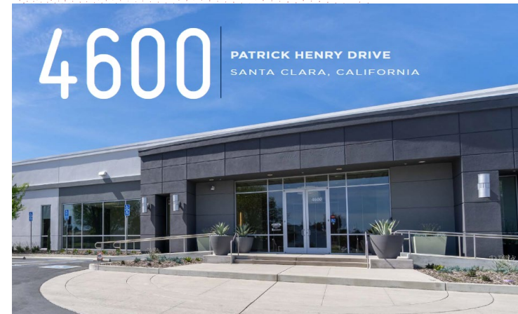
State-of-the-art facility in Santa Clara, California
